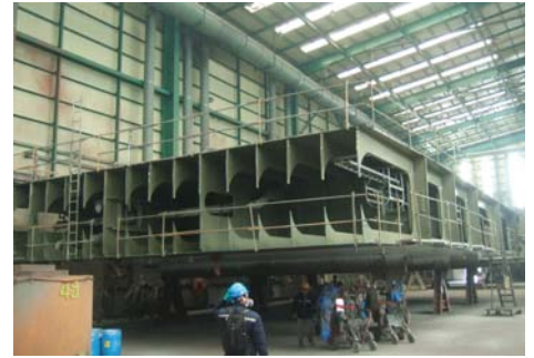
Intergard®7500 applied to a cofferdam
